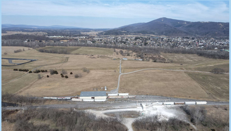
SITE OF FUTURE PVTA HYDROGEN FUEL PLANT
